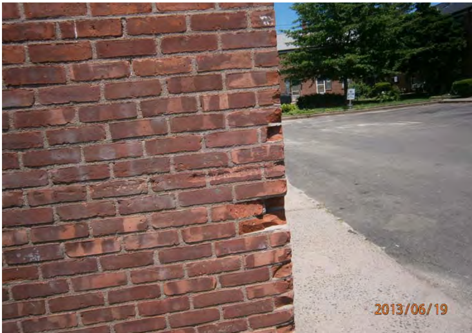
11. Building bricks, spalled
