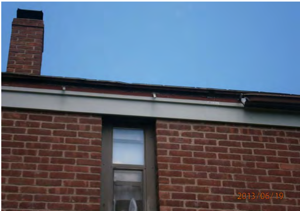
15. Gutter missing
