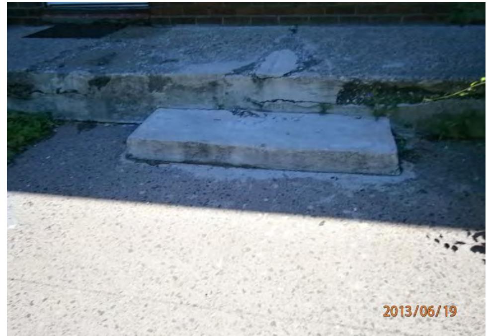
2. Damaged concrete pad
