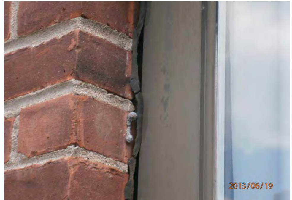
12. Caulking failures
