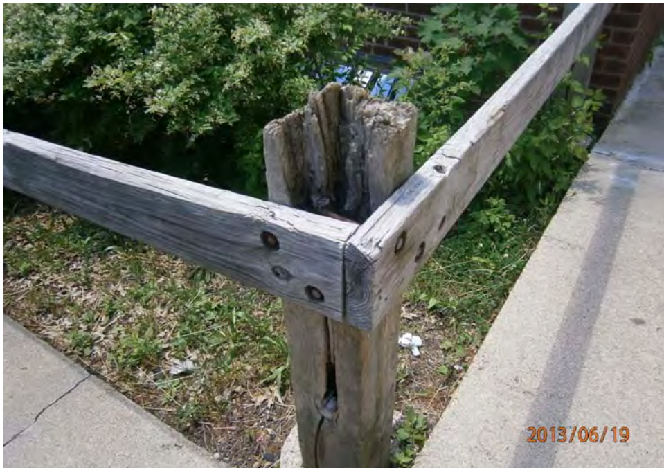
3. Walkway railing damage
