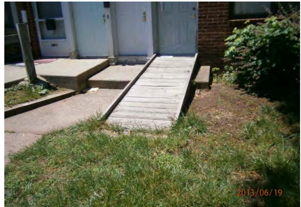
36. Accessibility ramp missing hand railing
