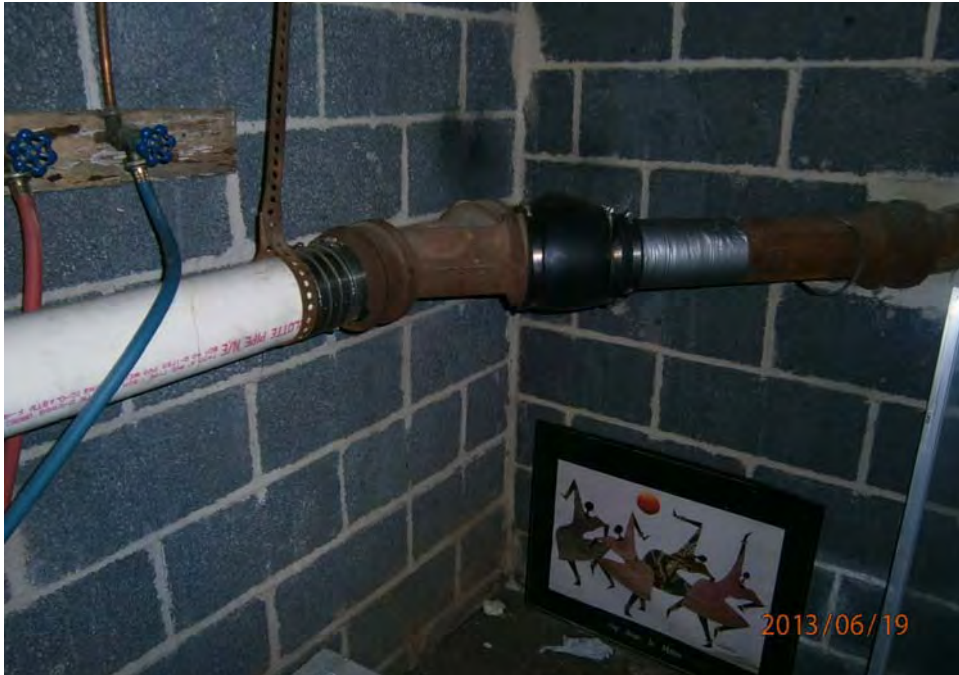
33. Typical unit waste line repairs
