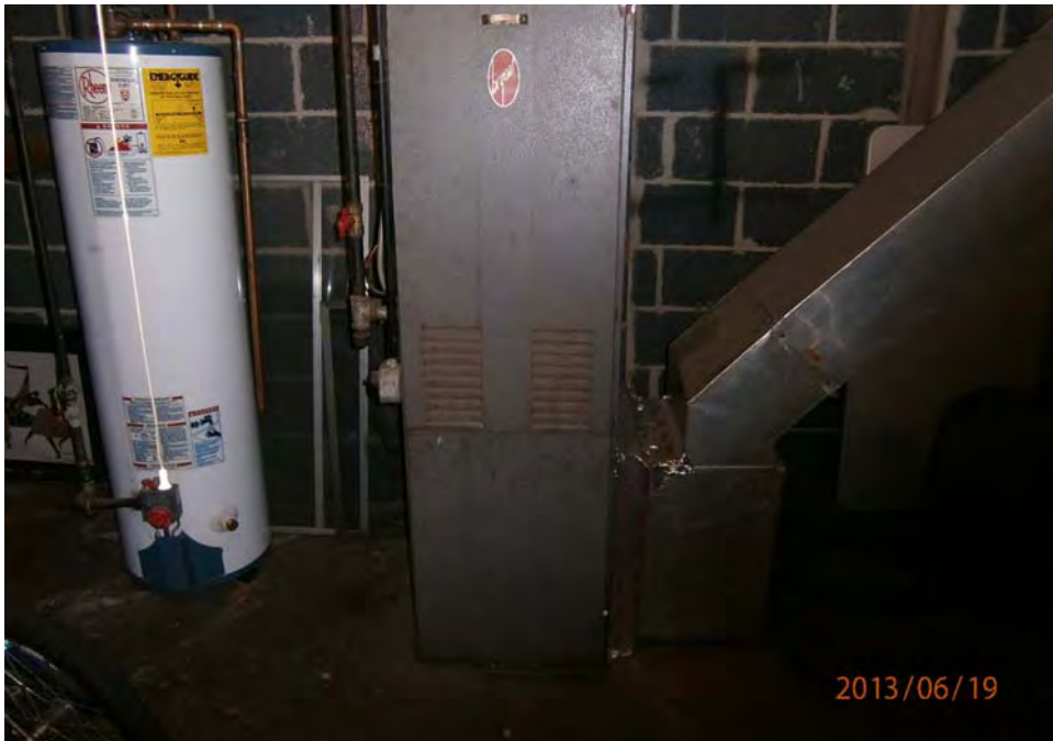
29. Typical gas furnace and DHW tank
