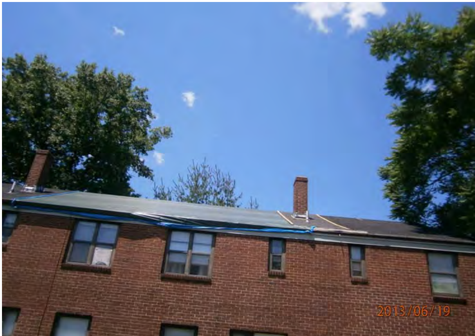
17. Temporary cover over damaged roof shingles
